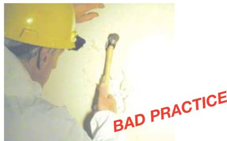
**Figure 5** Maintenance worker, working on asbestos insulating board without adequate controls
