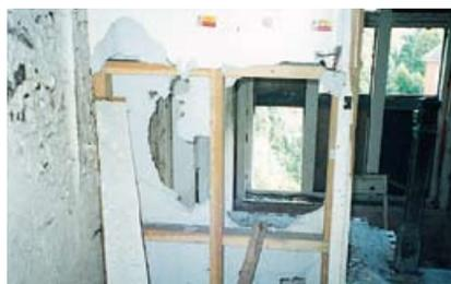
**Figure 7** Asbestos insulating board wall panels badly damaged
